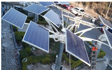
3KWp Solar Tree
